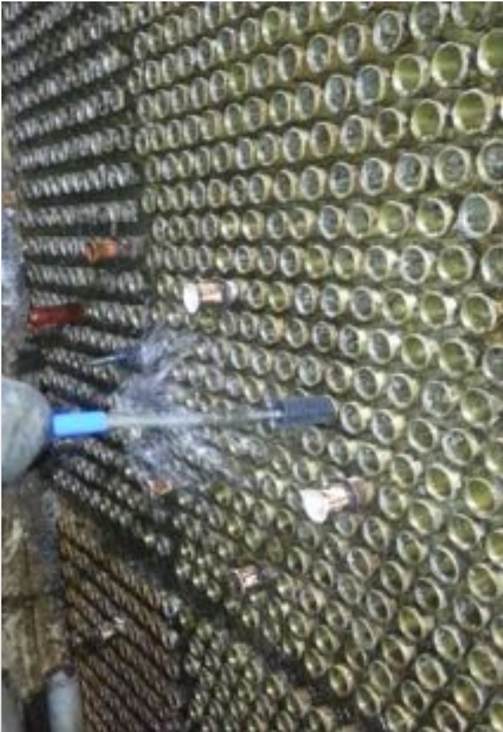
Copper alloy tubes in seawater
